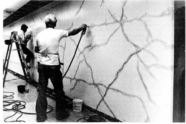
REPAIRING DAMAGE to corridor walls in Bldg. 912 are workmen from the Adhesive Engineering Co. Cracks created by the January earthquake are filled with epoxy from pressure gun. Quake damage was greatest in Bldgs. 912 and 911. This is the first phase of a Labs-wide rejuvenation, estimated to cost about \$400,000.
